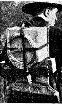
This portable radio set is an important part of the back pack of this member of the United States Forest Service. It is used in quick reporting and communication during fire emergencies in national forests. The two types of portable sets weigh 10 and 35 pounds and have average radii of 10 and 50 miles respectively.
