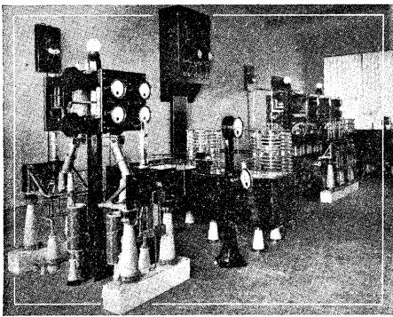
The new radio station is situated in the geographical centre of Europe, some 35 kilometres east of Prague, in the vicinity of the small town of Cesky-Brod. This new high-power broadcasting station is rated at 200 kilowatts (C.C.I.R.), and is the most powerful broadcaster operating in the medium wave broadcast band. The illustration shows: The power amplifier from the front, looking right, at the new Prague broadcasting station.
