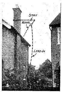
Fig. 4.—Supporting the aerial from a short stay fixed to a chimney.
