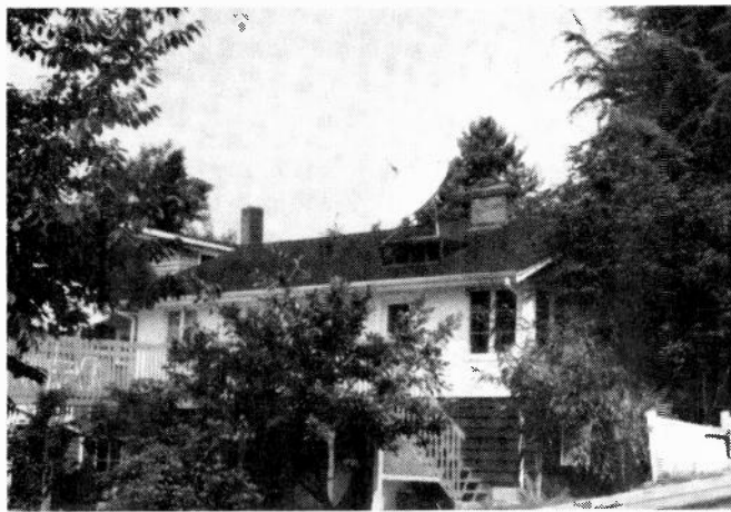
House in N. Vancouver, B.C., with roof-mounted dish aerial for satellite TV reception.
