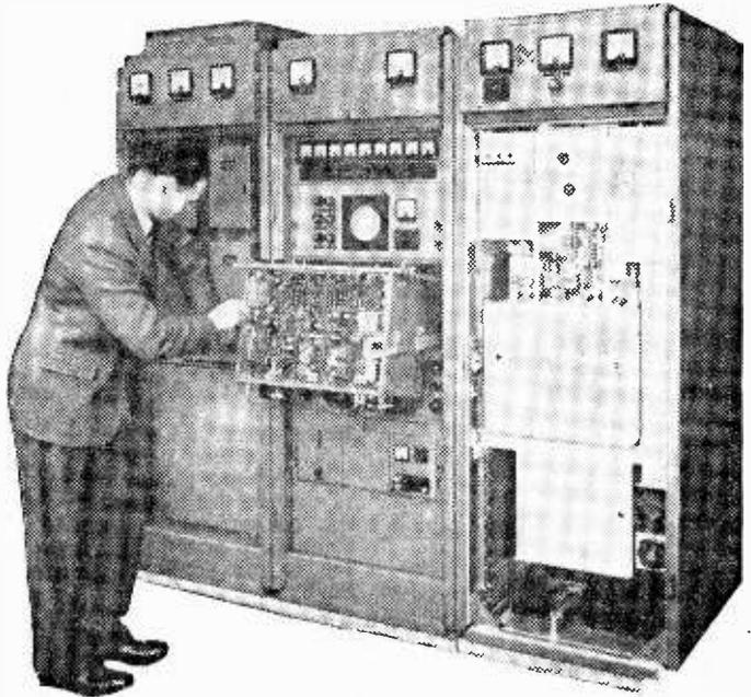
*A Marconi type BD 366A, 4kW vision transmitter under test at the Company's Chelmsford works. The front doors have been removed and the submodulator unit withdrawn for test purposes.*
