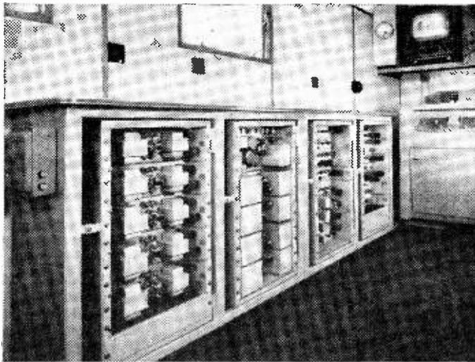
The first mobile Ampex Videotape recording unit to be mounted in a specially designed vehicle is being put into operation by TWW. The view above shows the interior of the van; all equipment is mounted in four low-level racks topped by a working area and in the background is the record monitor and part of the Ampex console.
