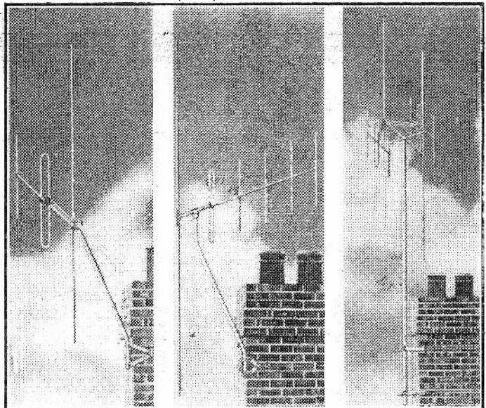
Fig. 18.—Photographs of some combined Band I and Band III aerials.
