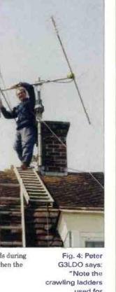
used for mounting the antenna ... don't even think about going on to a roof without these"1
