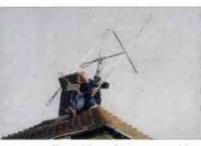
Fig. 2: The reflector assembly being fixed to the end of the boom.
