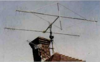
The antenna is mounted on a short mast on a KR-600RC rotator, which is fixed to the chimney using a double clamp. Some idea of the small size of the MQ-2 gain can be seen by comparison with the u.h.f. broadcast TV antenna.
