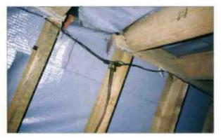
Fig. 3: Photo showing the centre feeder connection of the h.f. antenna. The conductor is supported to the timbers by a cord, while the helixes are wound on roof timbers insulated by a plastic membrane (but large diameter plastic piping could be used as an atternative).
