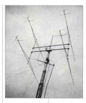
Fig. 1: The four 17-element 144MHz Yagi arrary used by David Butler G4ASR.
