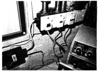
Individual mains plugs should be labelled with their functions using Dymo Tape or similar system. You will need several socket outlets
