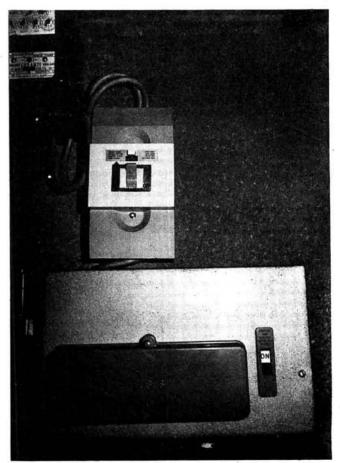
An Earth Leakage Circuit Breaker (e.l.c.b.) should be fitted between the meter and main consumer fuse box
