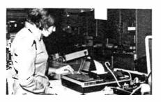
Signs of things to come. A complete data terminal in an attache case. It comprises a full keyboard, all necessary electronics, and a small collapsible television screen which folds down. The station may be used over a standard telephone via a modem, and can chat to computers and data terminals anywhere in the world
