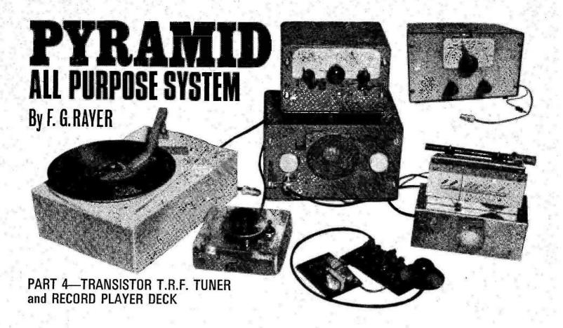
THEN the main need is reception of the stronger BBC transmissions, a t.r.f. tuner can give excellent results. Construction is much simpler than that of a superhet tuner, and the alignment difficulties sometimes experienced with the superhet circuit are absent.
