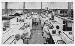
Part of a large clean room containing the integrated circuit diffusion centre. In our picture operators are loading and unloading diffusion furnaces.
