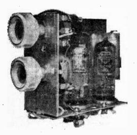
OW that ECL86 valves are easily obtainable it is possible to construct a useful portable record player for a reasonable sum. The ECL86 is a modern noval-based triode-pentode valve, the triode portion having an amplification factor of 100. The output pentode will deliver up to 4W of audio with an input of only 3'2V r.m.s. and because this is more than adequate for the use required, some losses due to tone control insertion can be afforded.
