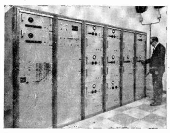
The new system has been installed by Standard Telephones and Cables Ltd. and includes about 200 reflex loudspeakers which are placed at key positions on the operating floor and which broadcast instructions to operating personnel from the control room. Staff can reply through a number of microphone units in the area; these are also connected to the loudspeaker network to enable other floor personnel to hear both instruction and reply.
