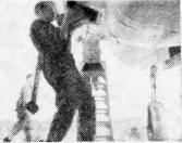
AS PART OF THEIR SERVICING. recharged batteries are hoisted into the Javelin's fuselage. These provide a reserve source of electric power.
