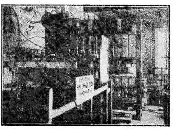
Some of the early apparatus at the Poldhu Wireless Station. On the extreme left are the transformers. The banks of condensers are carried in metal containers in the wooden rack. On the extreme right is the spark gap consisting of two steel spheres mounted on insulating rods. Used in sending first Trans-Atlantic signals, 12th December, 1901.
