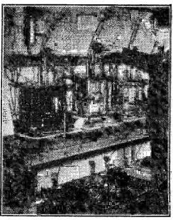
In this part of the G.P.O. Research Station water-soluble piezo-electric crystals are being "grown" in various solutions.
