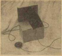
View of the complete receiver housed in a gas-mask box.
