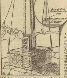
Method of mounting an aerial in a concrete block
