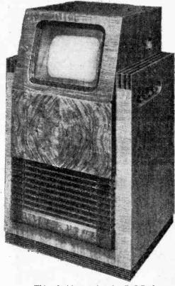
This television receiver by R.G.D. has a Thyratron time-base and employs magnetic scanning. It gives a toin, by &in, picture.
