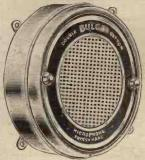
TWO carbon microphone elements arranged for push-pull operation, contained in a highly polished case which is substantially non-resonant. Sensitivity is
