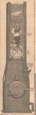
A training tank with latest type of escape lock, as built in new submarines in the British Navy.
