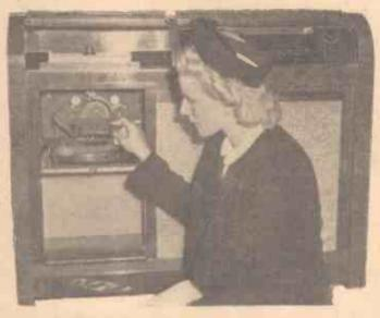
A feature of the Berlin Radio Show is a radio gram utilising a 24ft.—long film band on the surface of which the music to be reproduced is cut.
