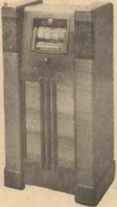
This view of the Pilot receiver shows the novel rotating full-vision dial which is a feature of the Pilot receivers.
