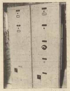
These are the two amplifier panels, the left one for broadcast and the right for television. At the bottom of each panel may be seen the time-control clock.
