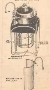
Fig. 3.—A popular type of Leclanche cell, and an alternative form of zinc plate.
