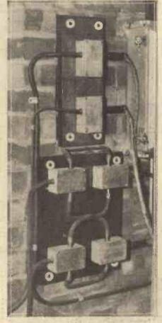
The output from each panel is fed to the single feeder through these distributor boxes.
