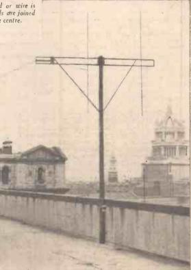
Fig. 3.—The method of leading off the feeder may be seen in this illustration of the aerial system used at the Science Museum, South Kensington.
