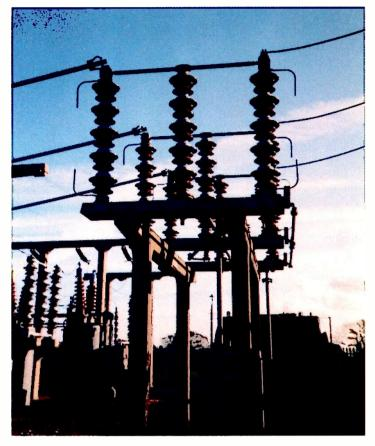
Arcing horns on a 33kV isolator.
