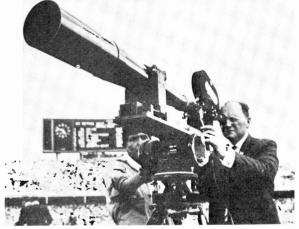
Film for TV: head close-ups at 500 ft. distance. A 1000 mm. Iens on an Arriflex (Techniscope) film camera in the centre of the Mexico Olympiad Sports Arena.
