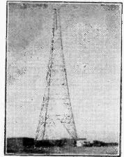
The aerial mast at Lichtield as it appeared when we went to press. The Marconi 16-stack aerial array is the first of its type to be designed and produced in this country.
