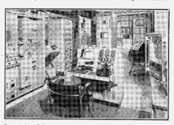
General view of the colour studio control room. On the left is the film scanner, on the right the power supply and pulse generator equipment. In the centre control console and three-tube colour picture monitor, and extreme right the radio check colour receiver.
