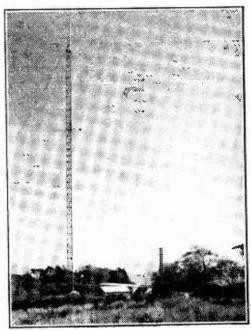
The 235ft, mast with 231ft, single-stack super turnstile aerial, horizontal polarisation, which Marconi's Wireless Telegraph Co. Ltd. erected at Glencairn Road, Belfast, in time for the Coronation.
