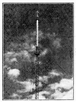
The slotted aerial at the top of the mast which is designed for use on V.H.F. sound broadcasting, should the BBC decide to adopt this system in the future.
