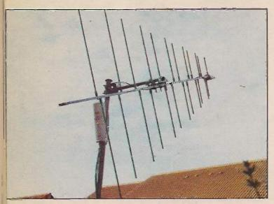
The Chelcom log-periodic VHF array Roger has been using for Fleetsatcom reception. The washing-up liquid container protects plug connections. A further plastic cover at the front of the array protects an encapsulated cable connection.
