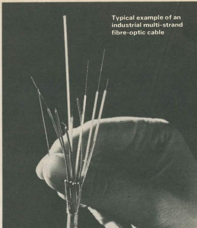
Typical example of an industrial multi-strand fibre-optic cable
