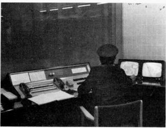
Local monitoring facilities are provided at Heathrow Central and platform-only monitoring of all three stations is provided for the line controller situated at Earls Court.
