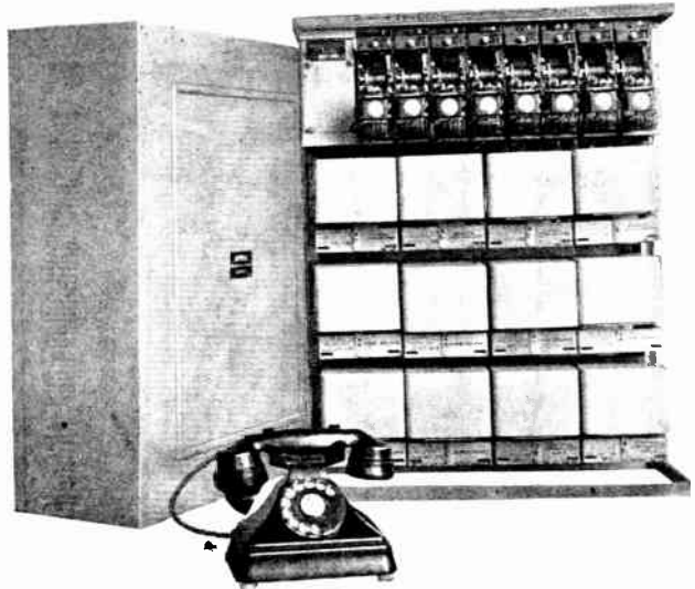
Fig. 12.—A SIEMENS 25-LINE RELAY TYPE PRIVATE AUTOMATIC EXCHANGE INCORPORATING THE "NEOPHONE" POST OFFICE PATTERN TELEPHONE. This is a 24-volt system.
