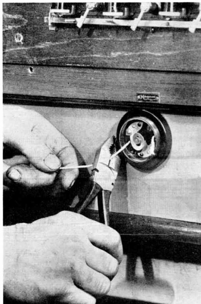
Fig. 37B. —CONNECTING UP THE PUSH. This shows the wires which come from under the indicator and through the back of the push being cut to the required length.
