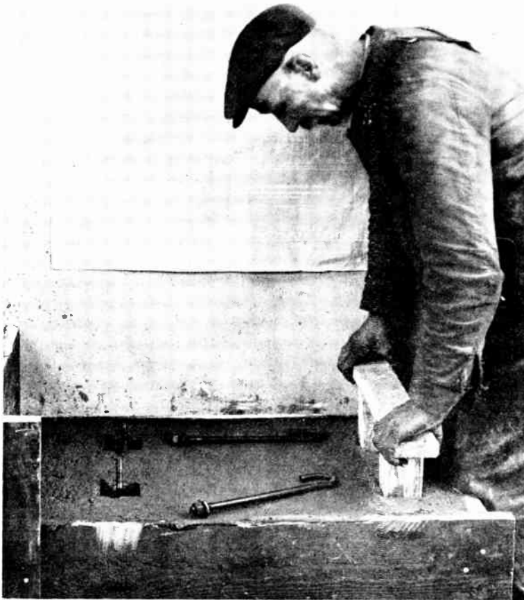
Fig. 2.—ANOTHER STAGE IN MAKING THE CONCRETE BED. (Stuart Turner, Ltd.)
