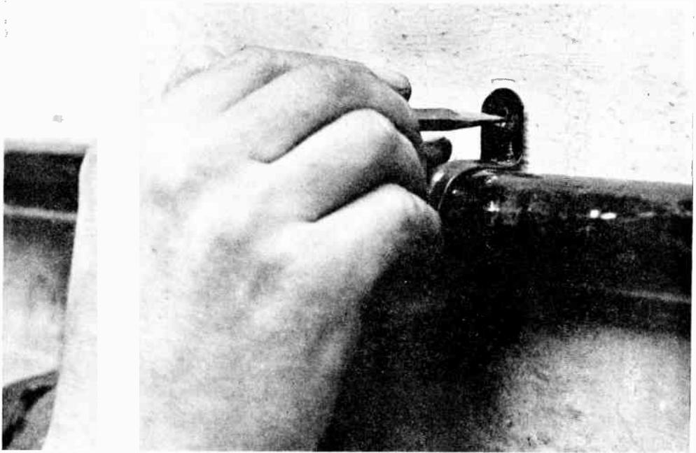
Fig. 7. —HOW TO FIX CONDUIT OR TUBING TO A WALL. FIRST OPERATION.
