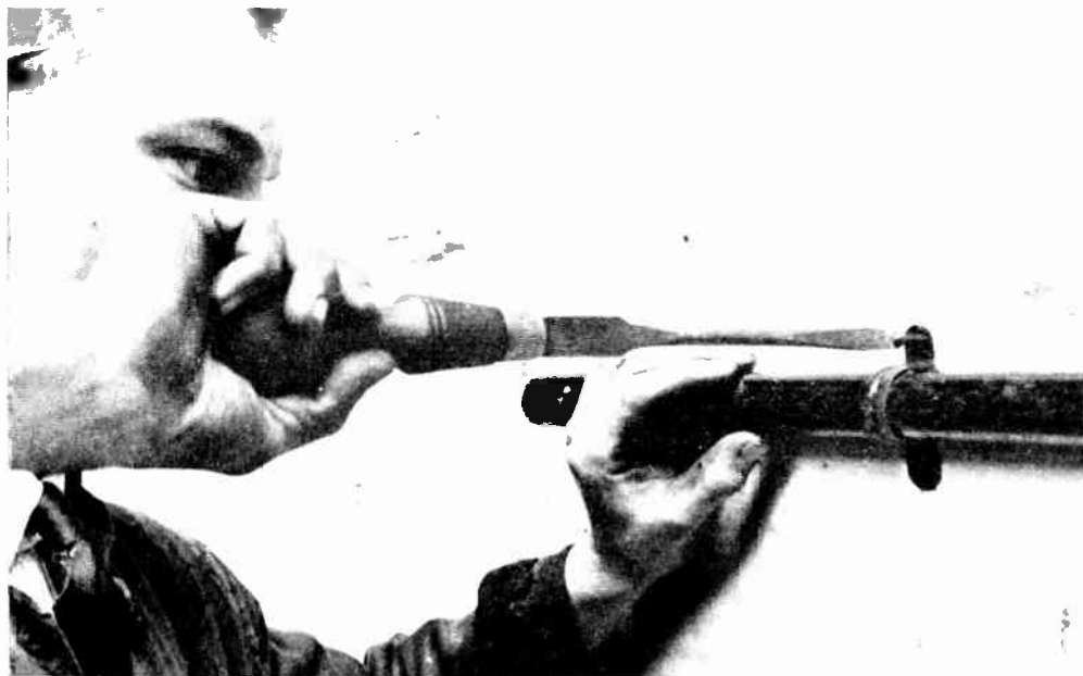
Fig. 10. —How to Fix Conduit or Tubing to a Wall. FINAL OPERATION. Screwing the fixing saddles in position.
