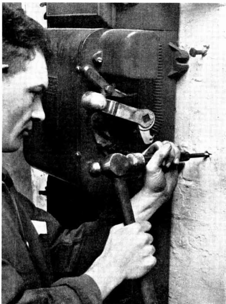
Fig. 1. —FIXING HEAVY SWITCHGEAR TO BRICK WALL. THE FIRST OPERATION.
