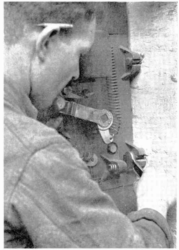
Fig. 3. —FIXING HEAVY SWITCHGEAR TO BRICK WALLS. THE FINAL OPERATION.
