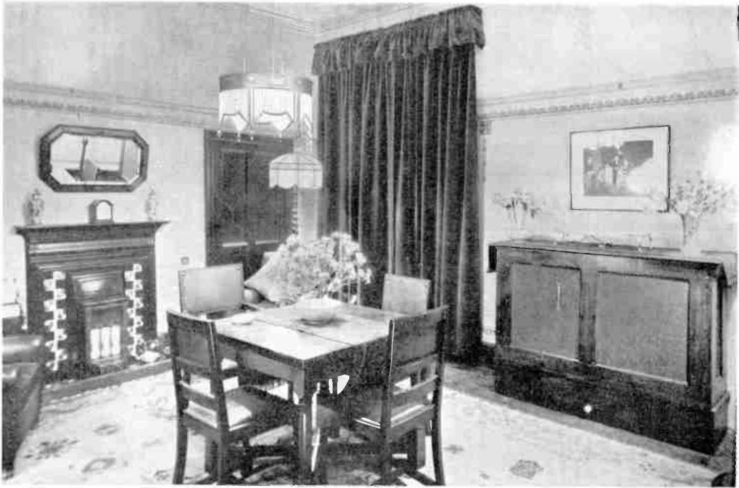
Fig. 9.—TYPICAL ARRANGEMENT OF LIGHTING IN A DINING-ROOM.
