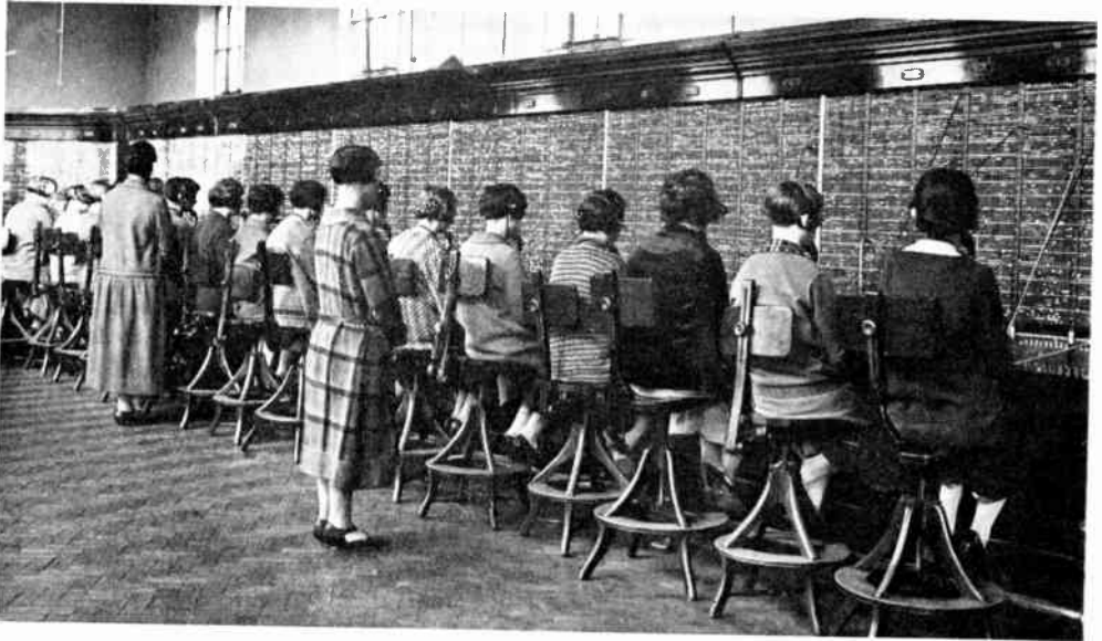
Fig. 1. —INSIDE A TYPICAL TELEPHONE EXCHANGE. This is a section of the Victoria Exchange switchboard, showing B positions with operators.
