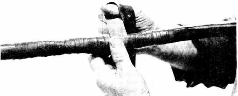
Fig. 5.—PREPARING C.T.S. CABLE FOR VULCANISING. Covering the joint with black tape.—(St. Helens Cable and Rubber Co., Ltd.)
