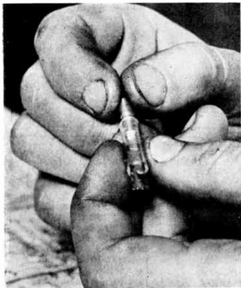
Fig. 1. —ASSEMBLING A GOLD FILM FUSE (1).
