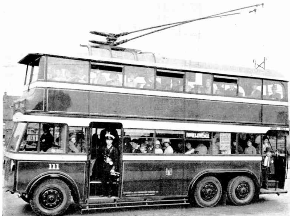
Fig. 2.—ONE OF THE LATEST SIX-WHEEL TROLLEY-BUSES. (English Electric Co.) The trolley-collectors are supported on a steel framework which is clear of the roof and is incorporated with the body framing
