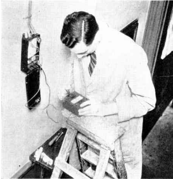
TEST TO EARTH ON A HOUSE INSTALLATION.
