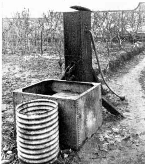
THE PUMP BEFORE CONVERSION TO ELECTRIC OPERATION. (B.T.H.)
