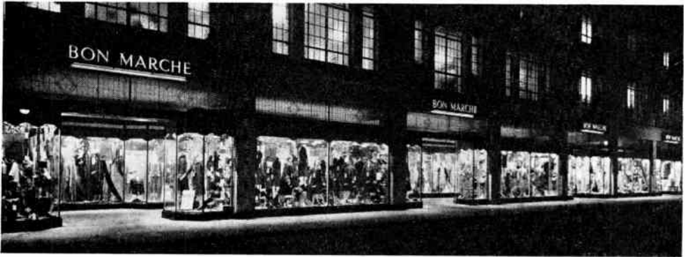
TYPICAL WINDOW LIGHTING WITH CONCEALED REFLECTORS.
