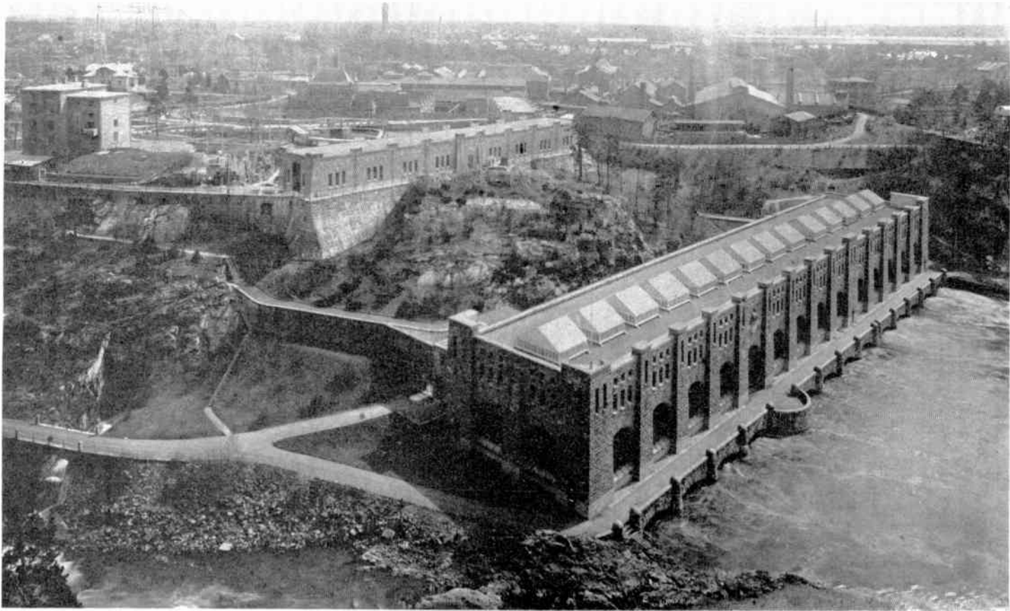
Fig. 4. —GENERAL VIEW OF TROLLHÄTTAN POWER PLANT.
