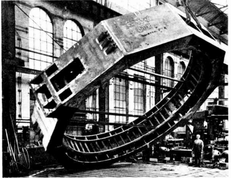
THE STATOR FRAME BEING TURNED OVER FOR COMPLETION OF WELDING.
