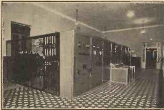
A general view of the transmitter at Bari. This station uses 20 kw., and works on a wavelength of 293.3 metres.
