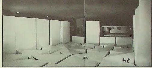
THE STUDIO interior with control room (left) and door to separation room (right). The wall and ceiling soundboxes were specially designed by Ken Shearer for Eden.
