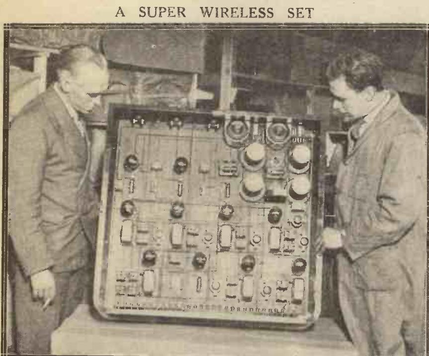
A huge wireless receiver made for St. Giles Hospital, Camberwell. It is designed to operate 550 pairs of 'phones and 42 loud speakers. The set is believed to be the largest in the country.
