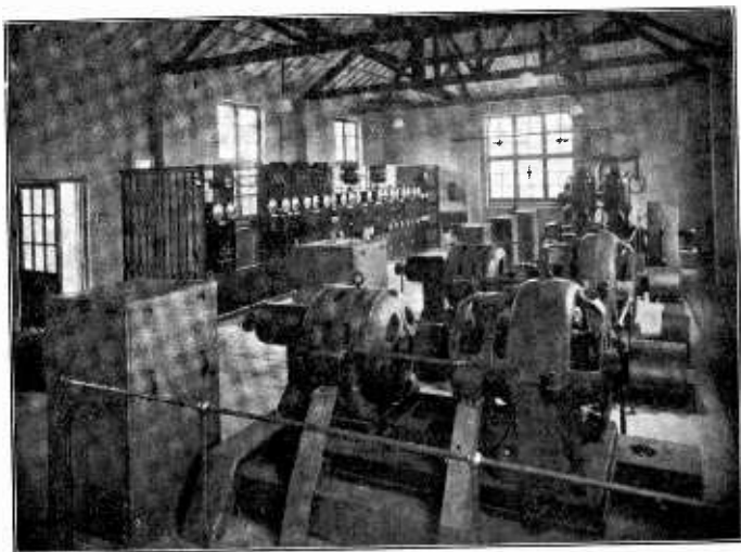
FIG. 2. THE POWER ROOM AT THE NORTHOLT STATION
