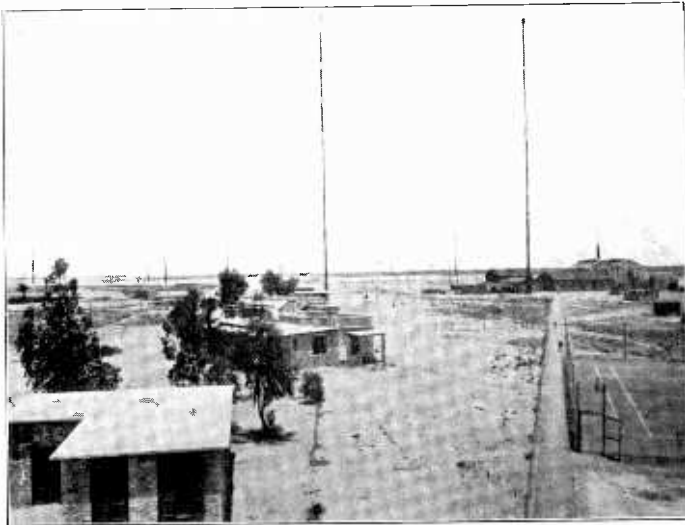
FIG. 5. THE HIGH POWER STATION AT CAIRO
