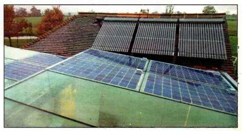
PV Solar panels and solar water collectors
