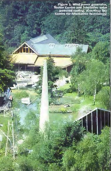
exported to the UK's National Grid. The completed on-site CAT solar roof covers an area of over 100 square metres, and should generate 9MW-hours of electricity each year, using pollution free solar energy (Figure 1).
