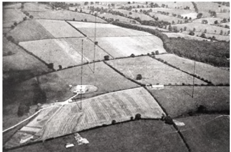
Positioned on Borough Hill, the BBC's Daventry transmission station has at various times radiated long-wave, medium-wave and short-wave broadcasts since it started operations in 1925.
