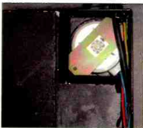
Expose the original motor.
