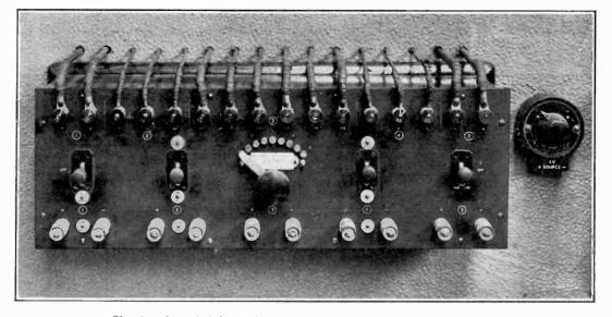
Showing the switch boxes for obtaining various supplies on the benches.
