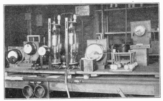
Fig. 6. Short-wave transmitter AGA.
