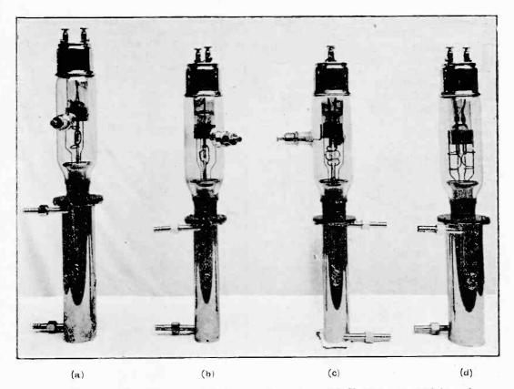
Fig. 5. Water-cooled values. (a and b) Transmitting values. (c) Short-wave transmitting value with two grid terminals. (d) Rectifier.
