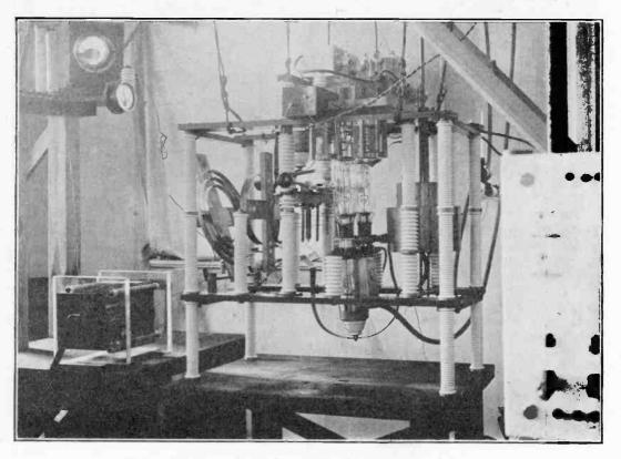
Fig. 11. Short-wave transmitter POW with two water-cooled values.
