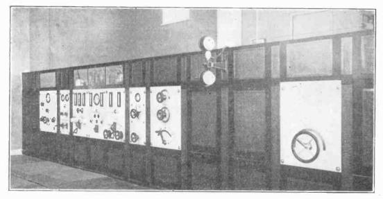
Fig. 5. Panels of the 14kW transmitter.
