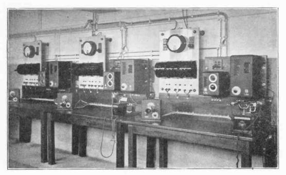
Fig. 2. The audio-amplifiers for the 7kW and the 14kW transmitters.
