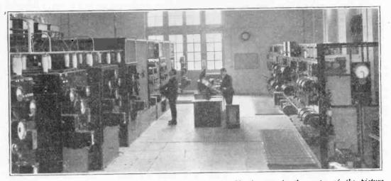
An internal view of the transmitting room. The control table is seen in the centre of the picture. The second engineer is standing beside the "excitation units," i.e., the 4kW and 50kW stages, as described in this abstract. To the extreme left are some of the power units. On the right is the L.T. switchboard.
