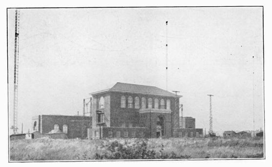
A general external view of the transmitting building. At the left-hand side of the building, on the upper window, can be seen the lead-in for the aerial now being used for the telegraphic transmission. The lead-in for the smaller aerial now being used for the experimental transatlantic telephony transmissions is at the corresponding window at the other end.
