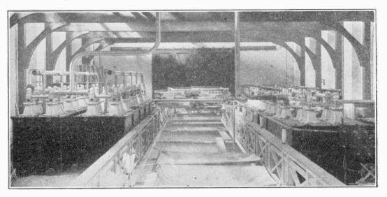
Mica condensers, oil-immersed, which are being used at the Rugby station. The mica pattern is much less bulky than the condensers of aluminium plates immersed in oil formerly designed by the Post Office for use at Leafield, and the adoption of the mica condenser has helped in the saving of space in the Rugby building.
