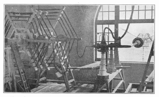
Photograph, taken from inside the building, showing the lead-in and also the inductance spiders.
