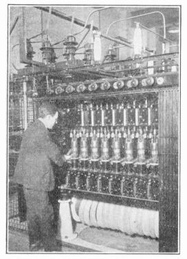
One of the power units with its Bostwick safety gate open on one side. The handles of the filament rheostat for each of the nine values forming one side of the unit are seen above the gates, while eight of the values are visible in the photograph, with an overload relay below each. The coil behind the insulator is a rubber water pipe.
