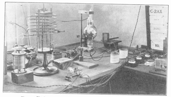
Fig. 19. The final amplifier and frequency doubling valve. The plate inductance and aerial coupling coil are shown on the left.
