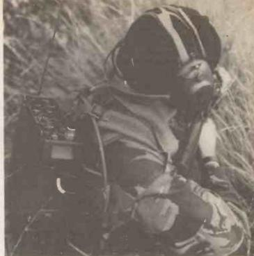
The **S**cimitar communications system made by Marconi is actually a family of several radio products, from pocket size up to vehicle-mounted systems. Digital data and voice communications can be transmitted on up to 284,000 channels and the system can automatically hop between channels at great speed to evade jamming.
