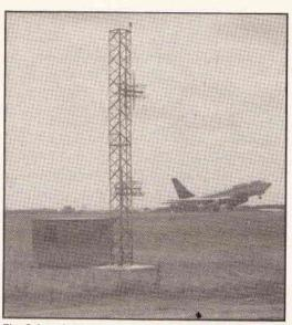
Fig. 8 A typical glide slope aerial. (Photograph courtesy of Racal).
