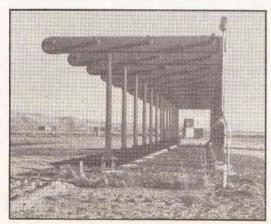
Fig. 7 An ILS localiser aerial, using multiple aerials to generate the azimuth beam. (Photograph courtesy of Racal).
