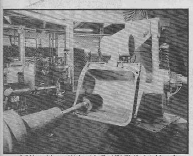
Polishing stainless steel kitchen sinks. The ASEA IRb-60 robot picks up the sinks and guides them against the buffing wheels which are attached to fixed spindles.
